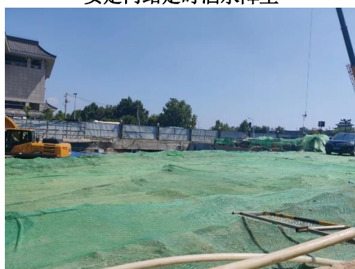
TJSG-14 标渣土遮盖
